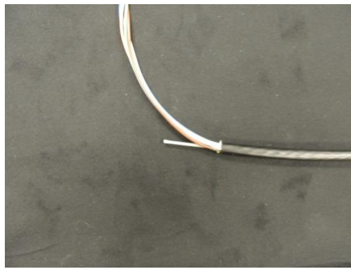
Leave approximately 5 cm (2 in) of FRP exposed to attach to the screw clamp inside the closure
